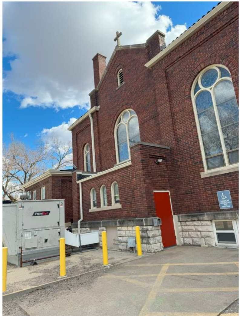
Figure 4. Existing Access Elevator Entrance
